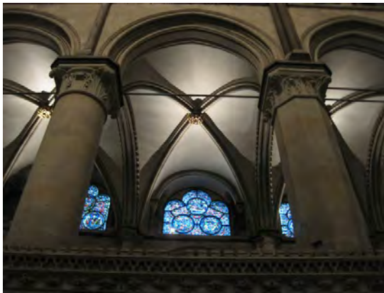
Fig. 12. Nave Vaulting Canterbury
